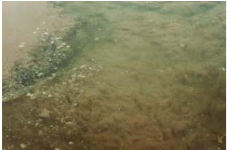
Fig 4. The activated sludge biomass begins to settle in the final clarifier. To maintain an optimal microbial population, part of the settled activated sludge from the clarifier is returned to the activated sludge basin, while another portion is wasted to prevent overpopulation.
