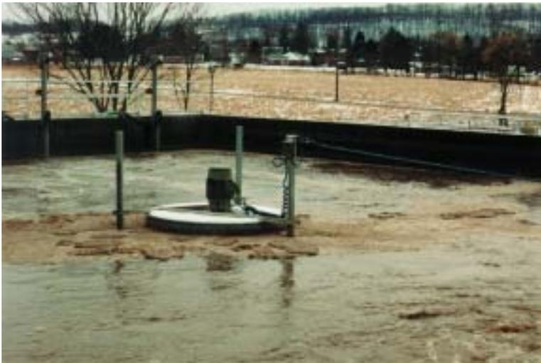
Fig 3. A floating mixer within the activated sludge basin keeps the biomass suspended.
