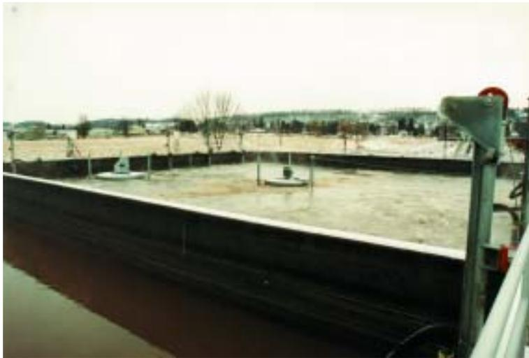
Fig 2. An activated sludge basin provides biological treatment of wastewater by providing conditions that encourage the proliferation of microorganisms that consume organic contaminants.
